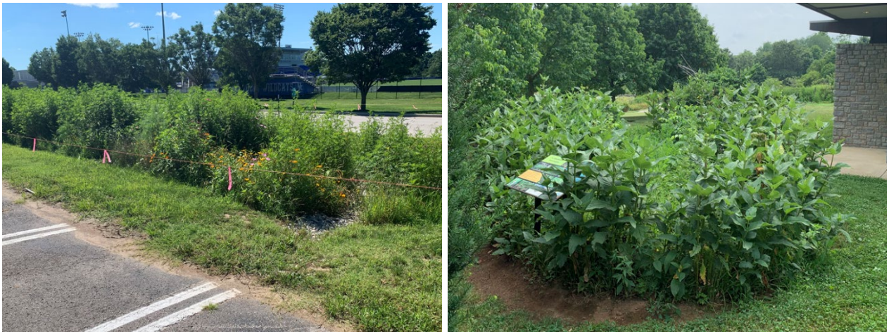
Figure 5.1–Wildcat Court Bioretention (left) and Arboretum Rain Garden (right)
