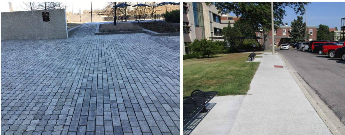
Figure 7.3—Garrigus Plaza Permeable Pavers (right) and Cancer Facility for Women Pervious Concrete (left)
