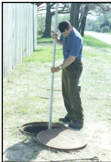
Sediment inspection using a stadia rod
